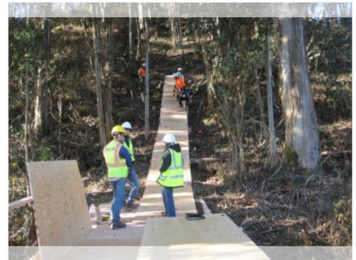
*SWCA constructed a ramp to skid vegetation over a creek without heavy equipment.*
